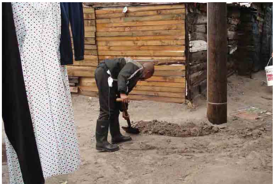
A man digs a channel to divert water away from the house
