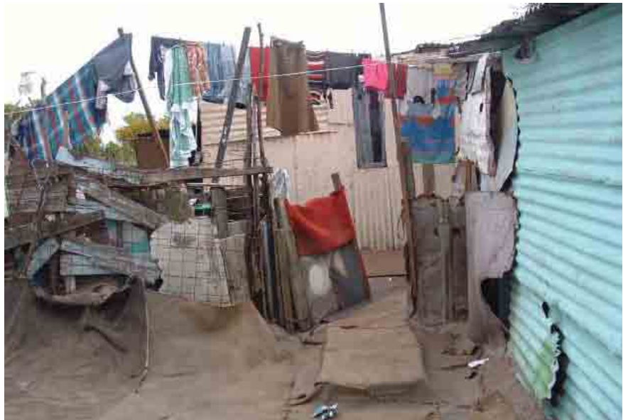
House elevated using a combination of sand and planking. The carpet covered step in the foreground leads to a raised interior.
