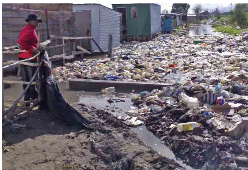
Waste blocks a water course
