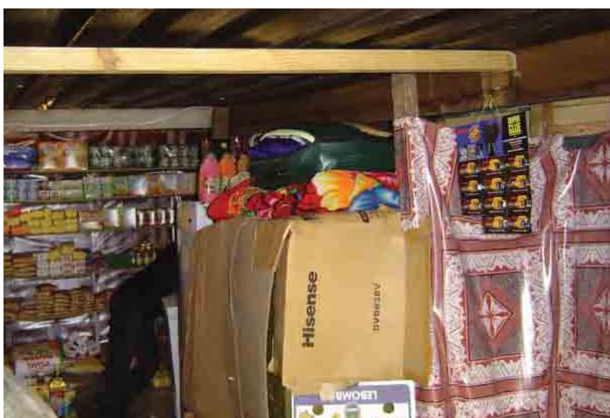
An electric sub-station concealed in cardboard in the middle of a spaza shop
