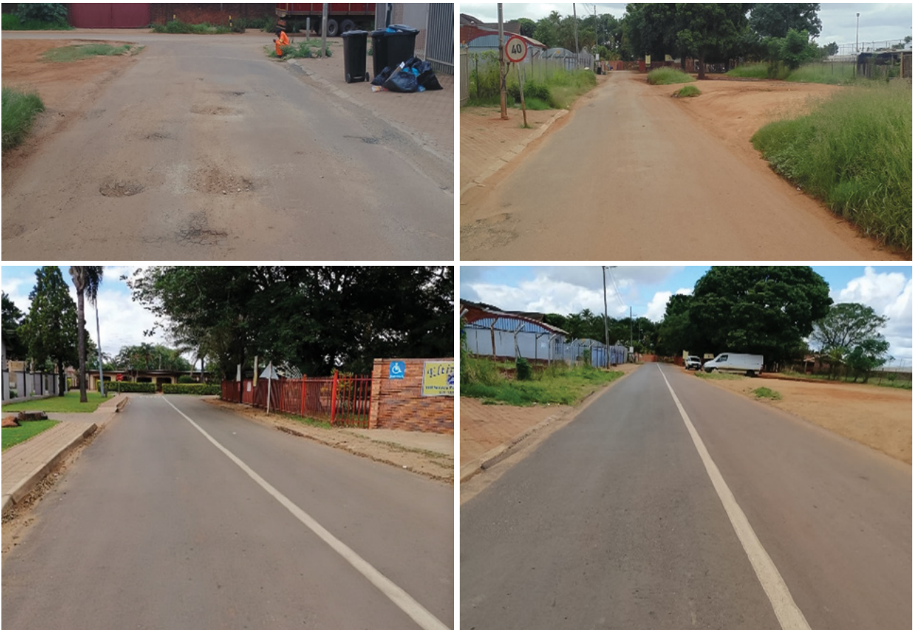
Figure 34: Eltivillas project before and after rehabilitation
