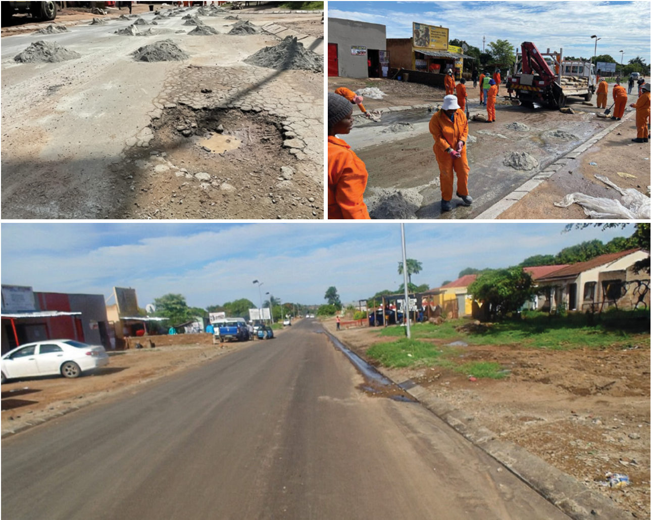
Figure 35: Malamulele section B and C during and after rehabilitation
