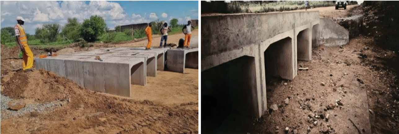
Figure 37: Makuleke culvert bridge during rehabilitation phase
