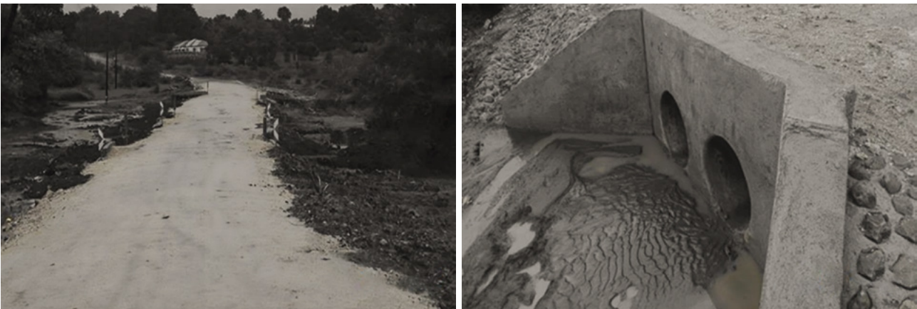
Figure 38: Tshikonelo gravel road rehabilitation
