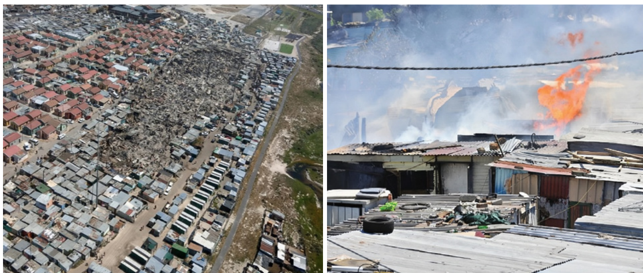
Figure 13: Non-compliance to building regulations in informal settlements
