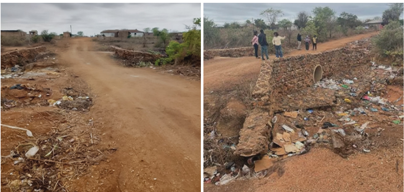
Figure 36: Makuleke culvert bridge project in Collins Chabane Local Municipality
